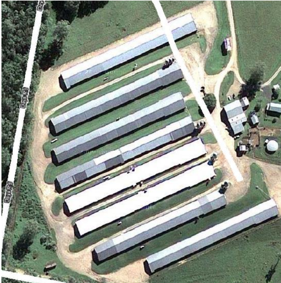
Figure 4-1: Aerial view of the Brisbane farm. The experiment was conducted in the bottom six sheds.
