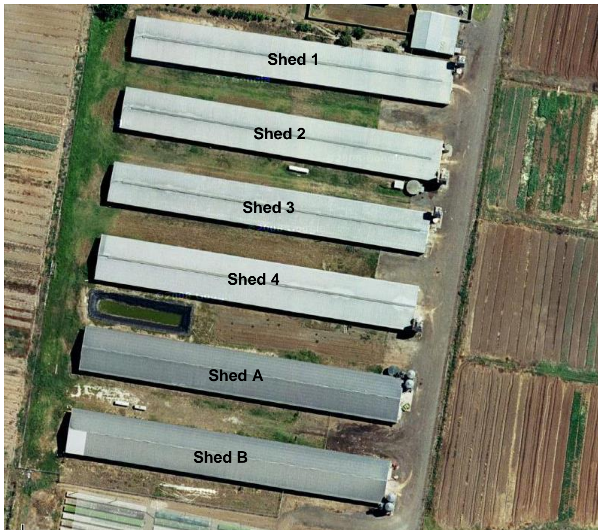
Figure 3-1: Aerial view of the broiler farm with sheds identified by name.
