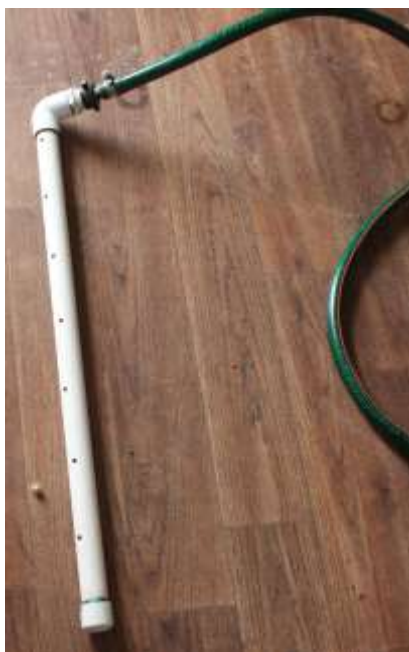
Photograph 13: Centralised Gas Delivery System
